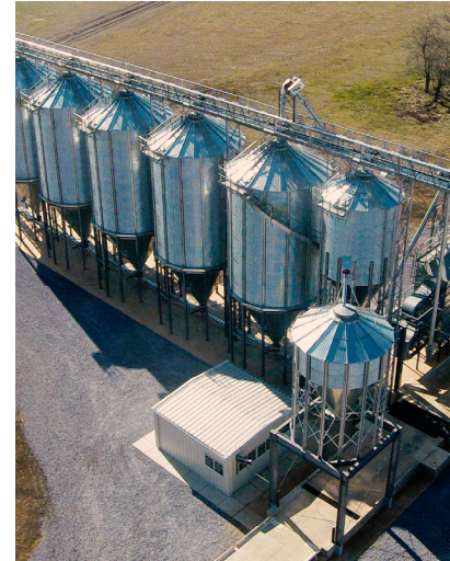
Installation of Grain Pump™ loop System with a wet bin and dryer application.
