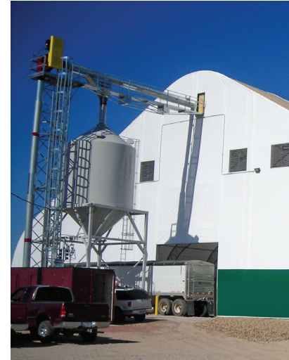
Installation of Commercial Grain Pump™ loop system into flat storage structure.
