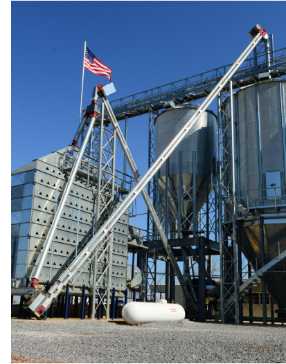
Stationary Double Run filling a dryer and unloading dryer to multiple bins.
