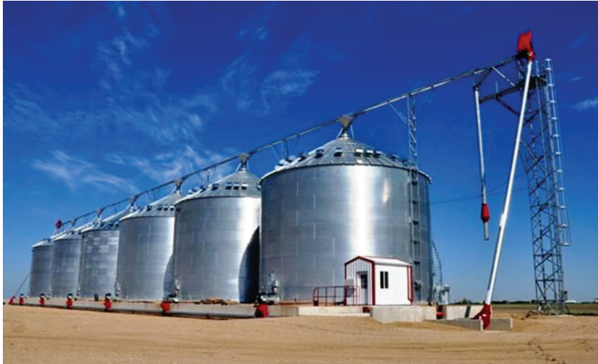
Installation of Grain Pump™ loop system into existing bin structure.
