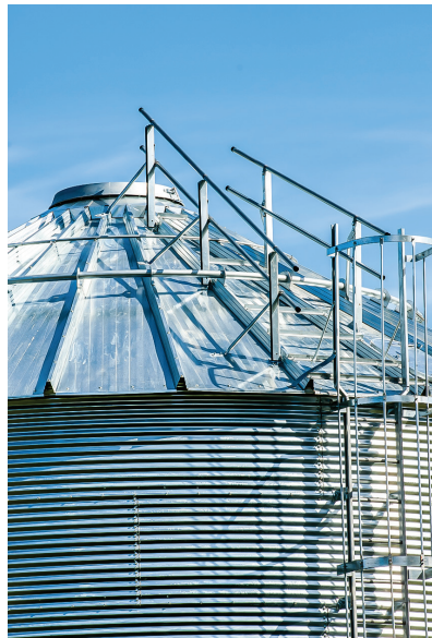
Roof Handrails
