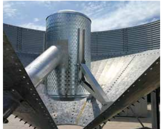
— Photo of hopper silo rocket aeration mounted on silo
