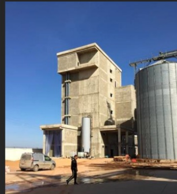
(Feed mill tower)
